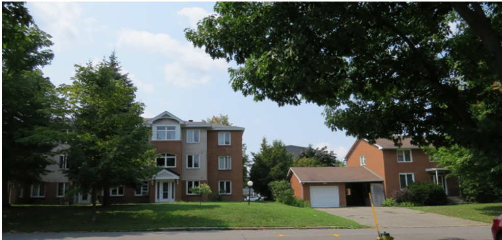
Ellwood House (left) and former St. Thomas rectory, 2270 and 2262 Braeside Avenue
